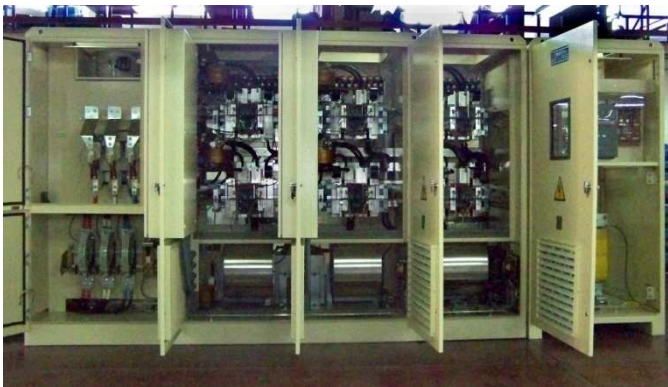
Fig. 18: Speed controller with IGCT for a 6.5 MW ball mill. By courtesy of International Electronics, Alcorcón, Madrid.
